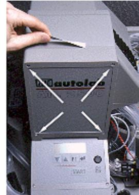
3. **IMPORTANT!** Label the location of the all wires plugged directly into the electronics head.
